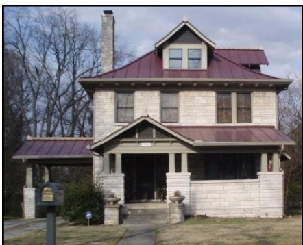
The residence at 1131 Greenfield is an exemplary illustration of an American Foursquare and one of just three in the district.
