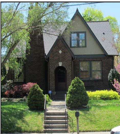
919 Caruthers is an example of a Tudor Revival style building.
