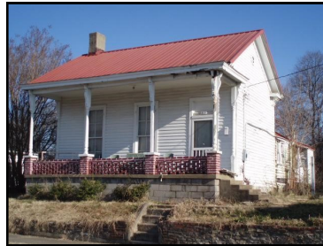
Side gable at 1810 5th Avenue North.
