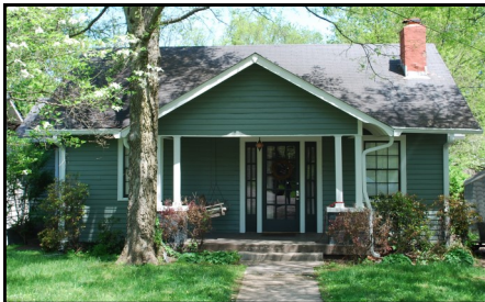
1127 McChesney is a good example of the bungalow form.
