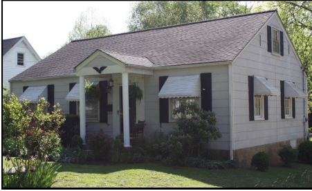
3518 Kennedy is an example of the Colonial Revival style applied to a Minimal Traditional residence.
