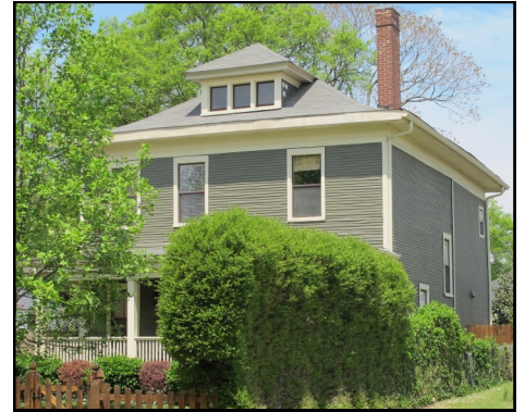
The majority of the homes are one and one-half stories, with the exception of just five two story homes, including this one at 920 Montrose.
