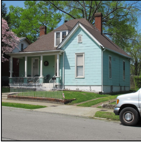
912 Gilmore is a Victorian-era building.
