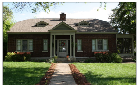
The Colonial Revival style is most often applied to modest homes of minimal scale, such as this one 1141 Greenfield.
