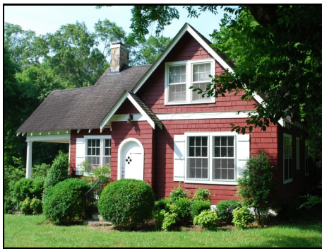
1402 Riverwood Drive is one of a handful of homes that does not have brick siding. It is an English Cottage style.
