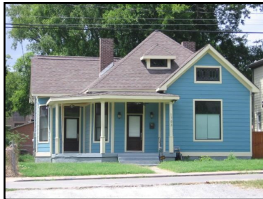
Cross gable at 1703 5th Avenue North.
