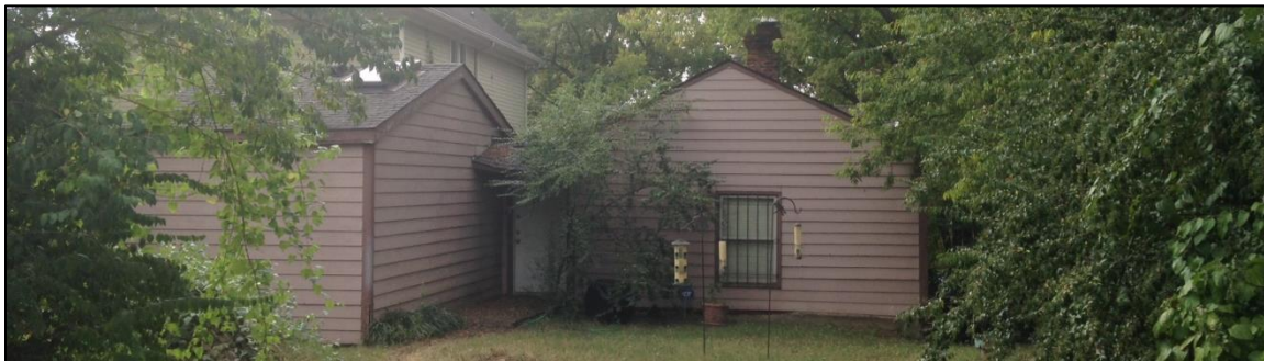
Figure 7 is a view of the existing addition from the rear yard.
