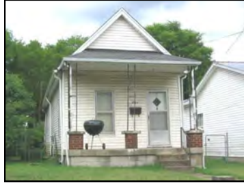
Shotgun with front porch at 1714 4th Avenue North.
