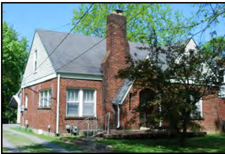
2312 Riverside Drive is a one and one-half story English Cottage constructed c. 1935.
