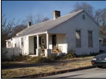
Shotgun with side porch at 1809 5th Avenue North..
