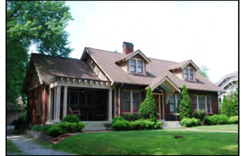
1104 Riverwood is an exemplary example of a Craftsman style bungalow in the Eastdale Place district.
