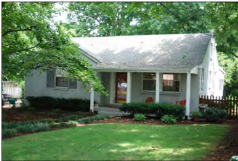
194 Kenner Avenue is an example of a Minimal Traditional.
