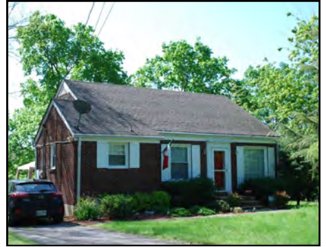
3504 Golf Street is a good example of a Minimal Traditional form.
