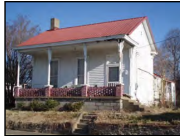
Side gable at 1810 5th Avenue North.
