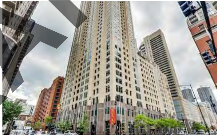
Appropriate upper level facade treatment with natural ventilation integrated into the facade design
