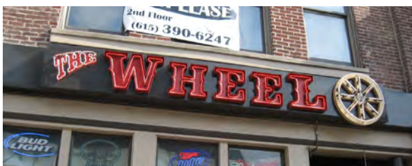
Example of raceway incorporated as sign background
