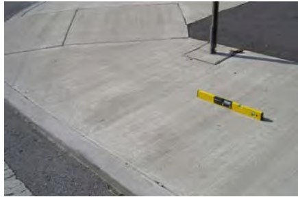
Approach Ramp Measurement (right)
