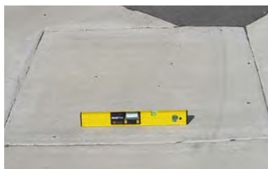
Reading 1: Front of Landing
