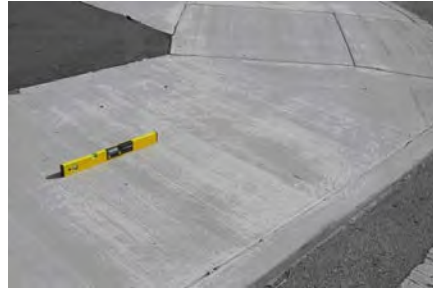
Approach Ramp Measurement (left)
