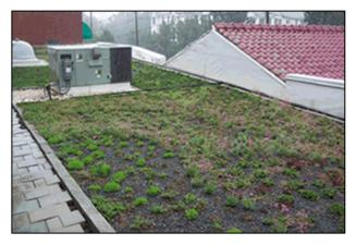
**Description:** A vegetated roof cover composed of hardy plants growing in an engineered plant medium, filter cloth, drainage layer, and waterproofing membrane. Green roofs provide benefits such as reducing runoff volume and peak discharge rate, reducing building cooling costs, and prolonging roof life.
