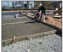
a mixture of open-graded aggregate, which creates the voids in the structure, and Portland cement. The void space in porous concrete is in the 15%-22% range compared to 3%-5% for conventional pavements. Porous concrete is thought to have a greater ability than porous asphalt to maintain its porosity in hot weather. The permeable surface of porous concrete is typically installed as the top of several permeable layers, similar to the installation of porous asphalt described above.
