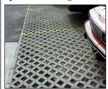
are structural units, such as concrete blocks or bricks with regularly interdispersed voids that penetrate their entire thickness. Grids are made of concrete or brick and the open cells are filled with porous aggregate or vegetated soil. Block pavers are more rigid and therefore can bear larger traffic loads than plastic grid systems.
