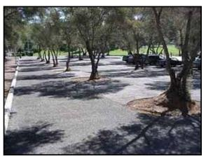
**Description:** Infiltration practices that are alternatives to traditional asphalt and concrete surfaces. Stormwater runoff is infiltrated into the ground through a permeable layer of pavement or other stabilized permeable surface.
