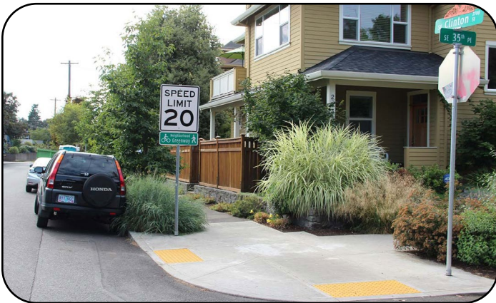
ADA ramps and corner landscaping
