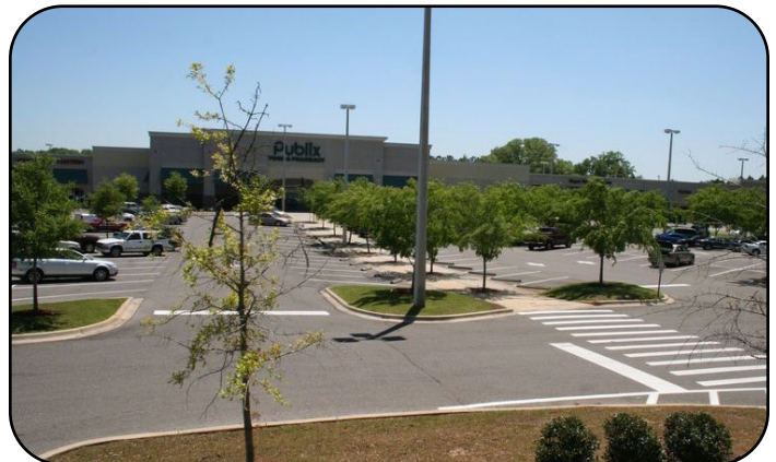
Pedestrian access through parking lots
