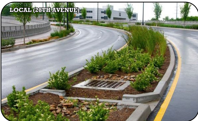
Integrated into crosswalk curb extensions
