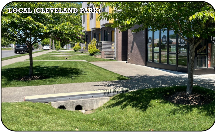
Stormwater management underneath sidewalk
