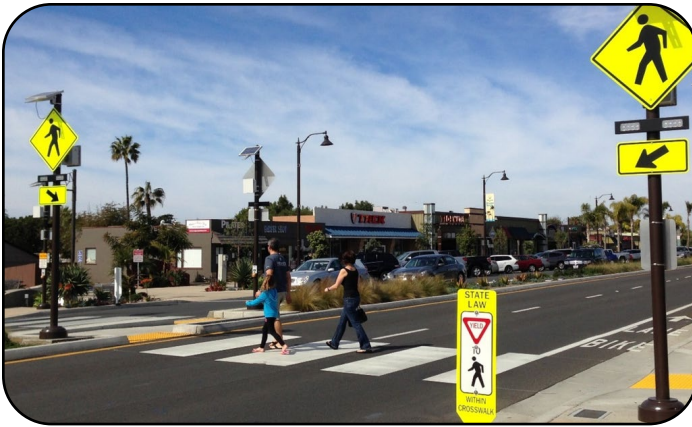
Rectangular Rapid Flashing Beacon (RRFB) activated by button
