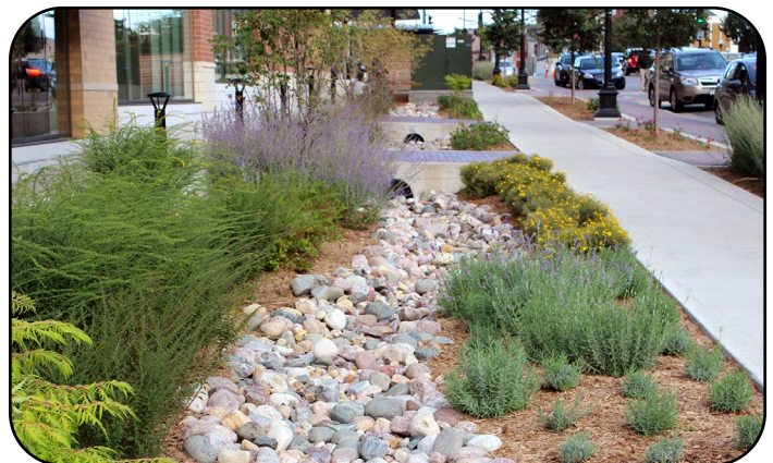
Stormwater management system
