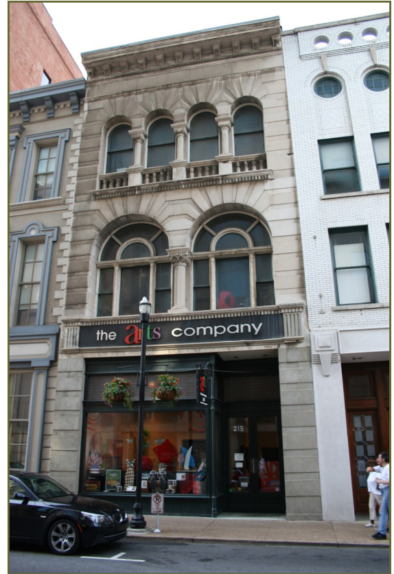
Original and early display windows like this at 213 Fifth Avenue North should be retained and, if needed, repaired using materials that preserve their historic appearance.
