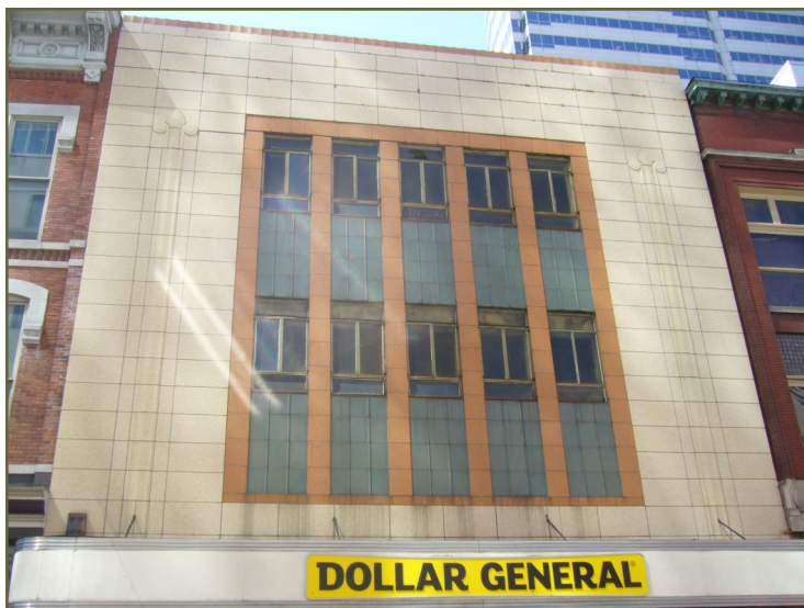
Window styles and materials downtown vary from single and double-hung windows, to metal windows of a more industrial design.
