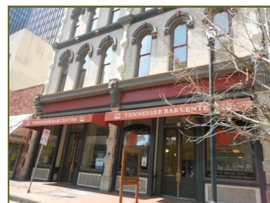
221 Fourth Avenue North was constructed in 1871 in the Italianate Commercial Style. While the storefronts have been altered, the façade retains its original upper floor details.
