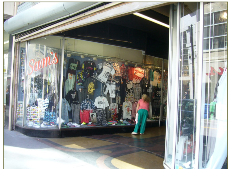
Several storefronts on Fifth Avenue North and in the Arcade have curved glass store fronts with deeply recessed entrances.
