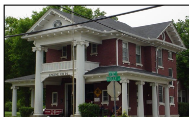
Holly Street Fire Hall
