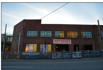
G.P. Rose and G&S Distributing Building
