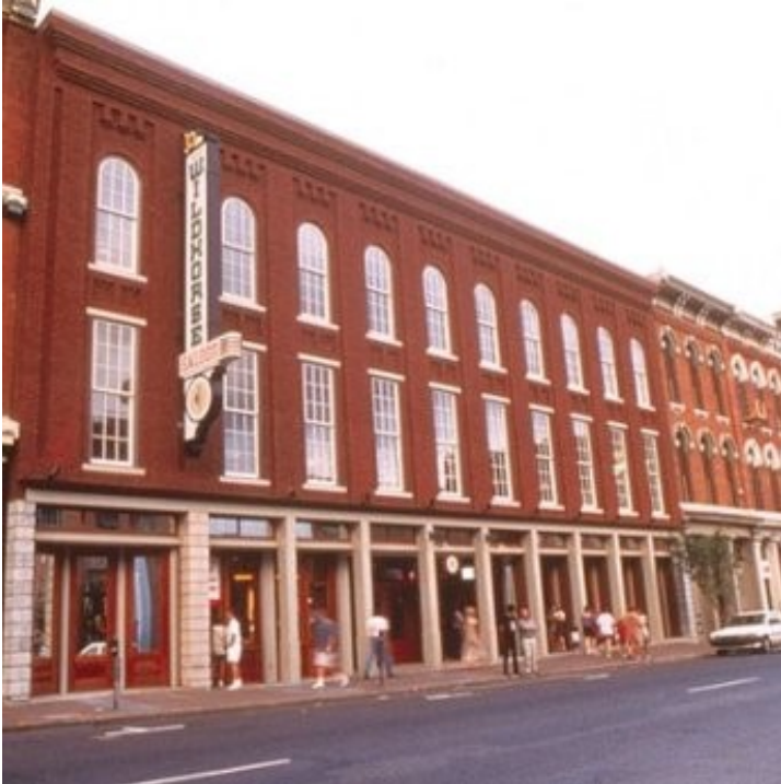
This building was reconstructed based on photographs.
