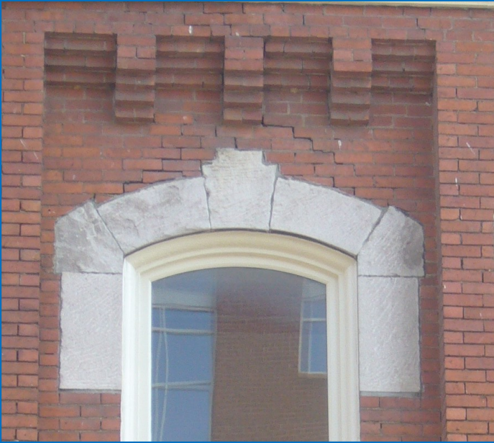
Decorative brick corbelling frames this window.
