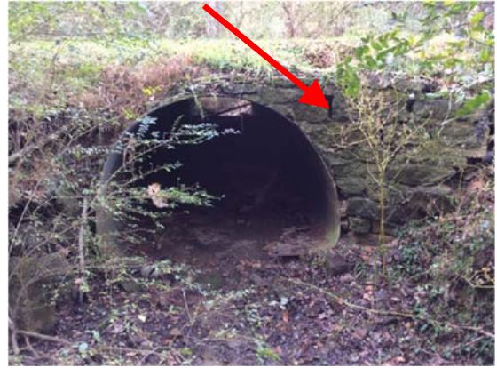
Failing Headwall
