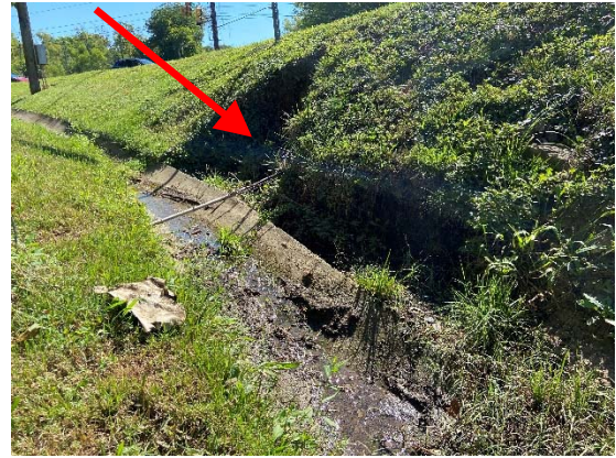
Embankment Erosion
