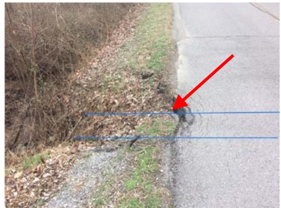
Pavement Failure/Settlement
