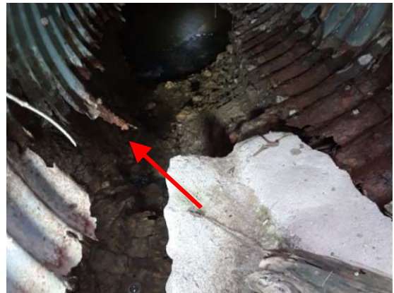
Failing Outlet Headwall w/ Erosion
