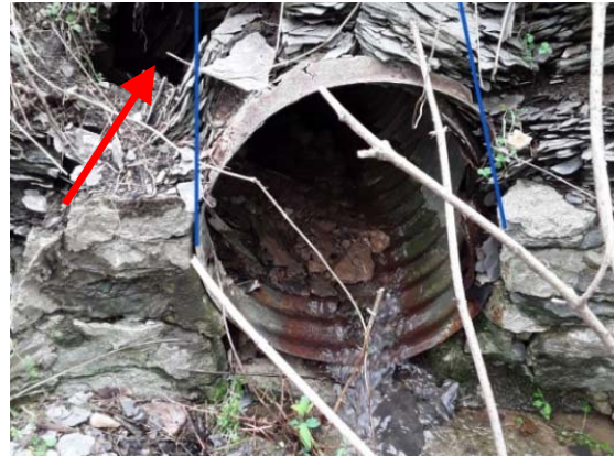
Failing Outlet Headwall w/ Erosion
