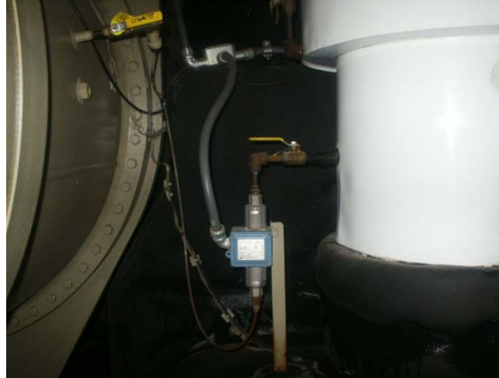
Differential Pressure Switch Isolation Valve (evaporator)
