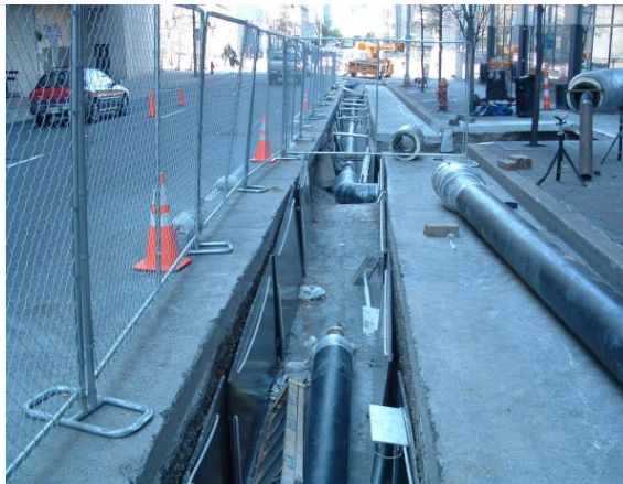
Manhole 5 to 9 Condensate Line Replacement
