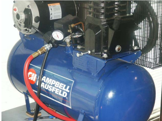
Plant Fire System Air Compressor
