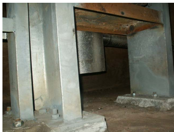
Manhole 1 Structural Steel Repairs
