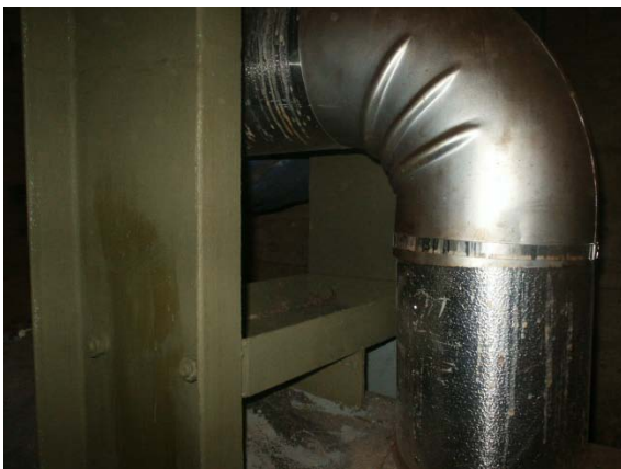
Manhole 1 Insulation
