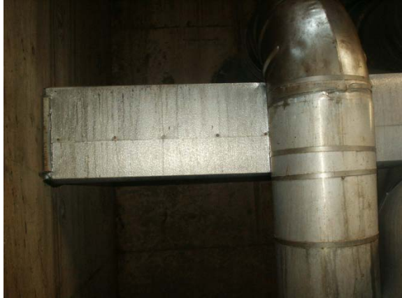
Manhole 5 Structural Steel Insulation
