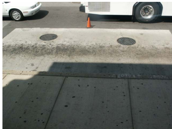
Manhole 10 Concrete Pad
