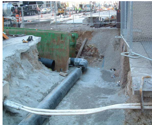
Manhole 5 to 9 Condensate Line Replacement
