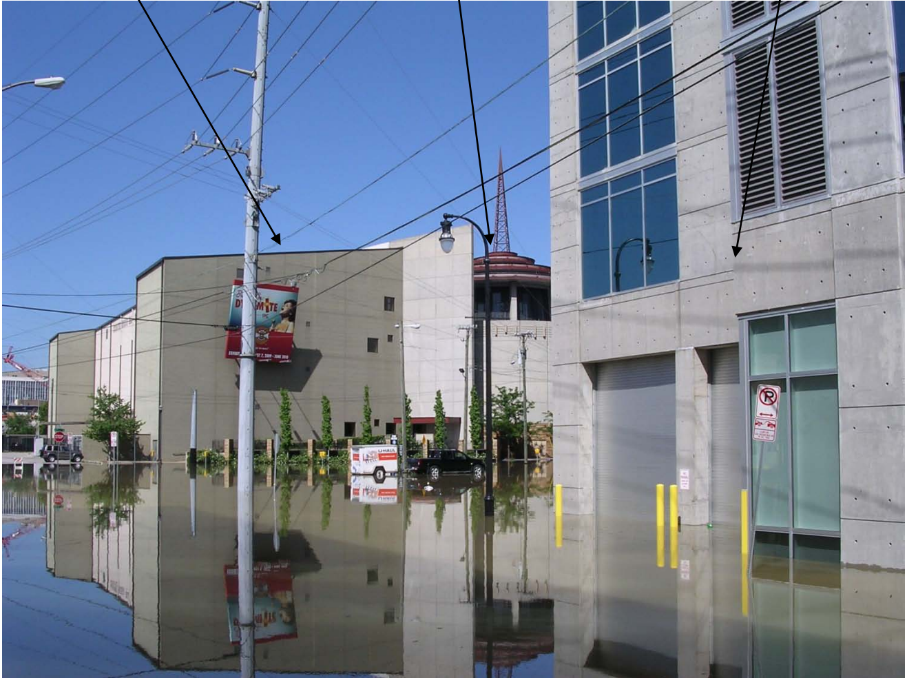
View of Malloy Street from 3 rd Avenue to 4 th Avenue
