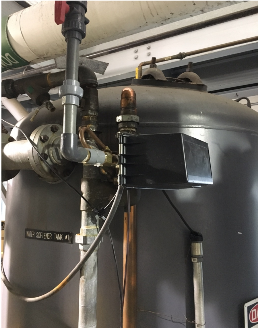
Controller upgraded on #1 Softener
