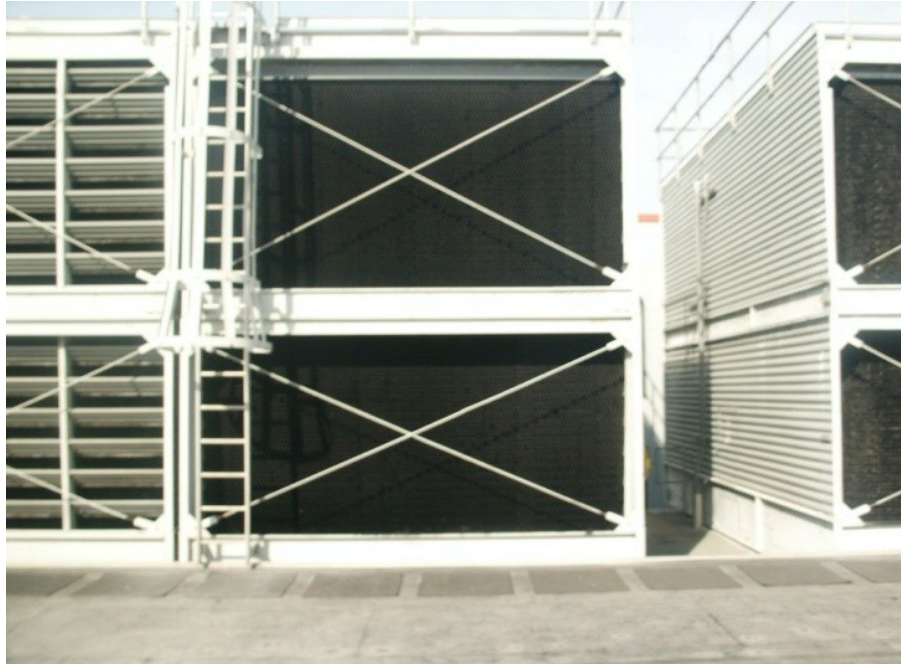
Installed new fill in #7, #8 and #17 Cooling Towers
