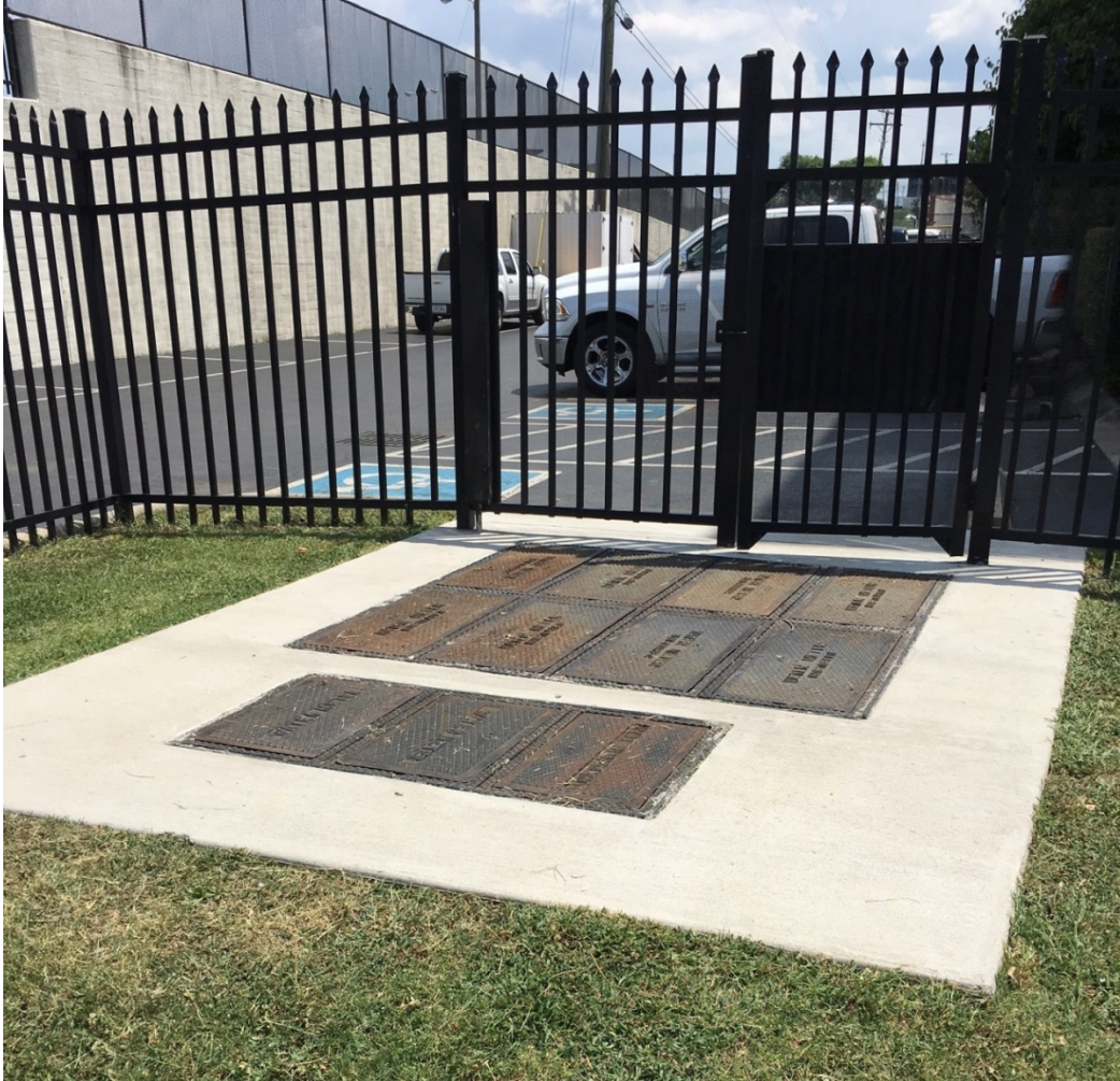
Added concrete pad around water meter boxes
