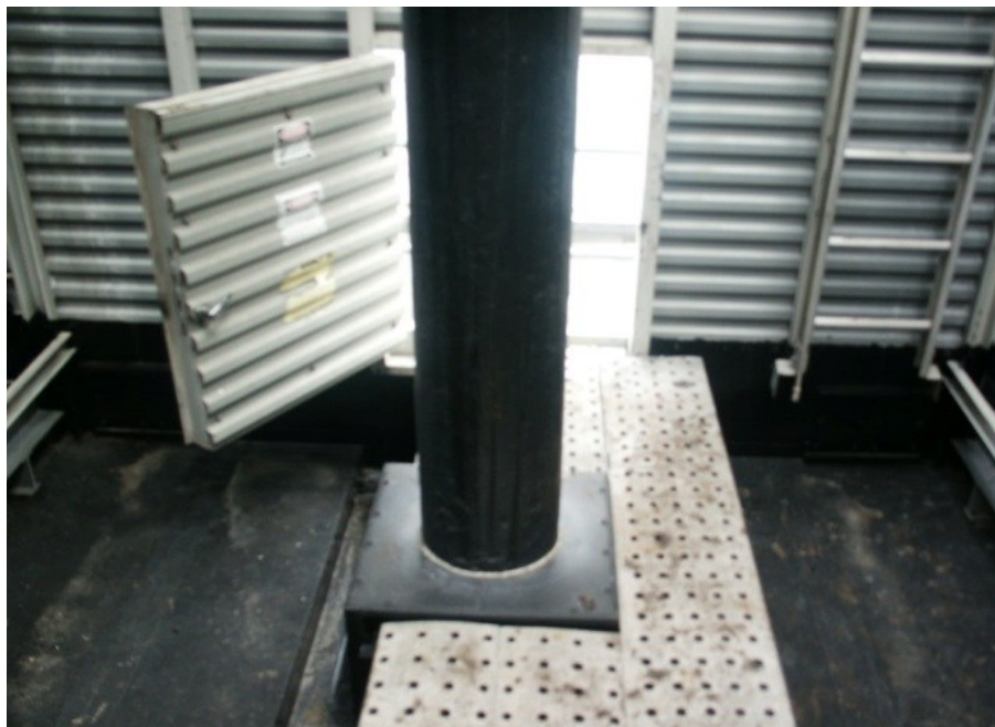
Re-coated the basins and riser pipes in #7, #8 and #17 Cooling Towers
