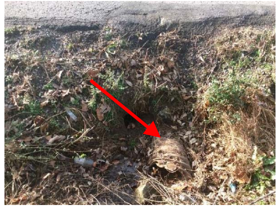
Crushed Pipe Inlet
