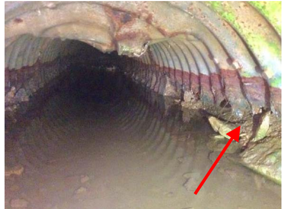
Crushed Pipe Inlet
