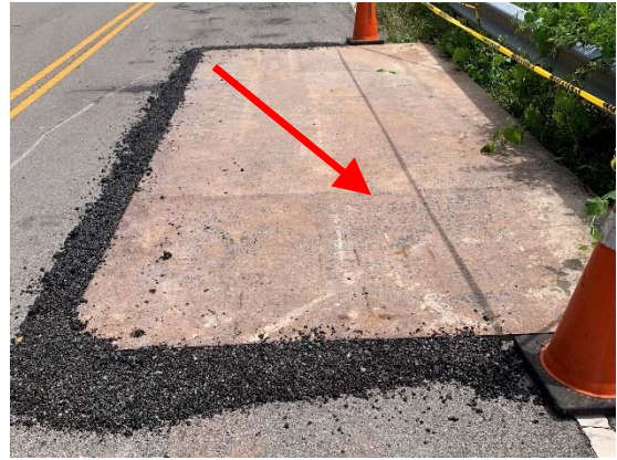
Roadway Failure w/ Steel Road Plate
