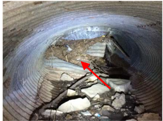
Failing Inlet Headwall
