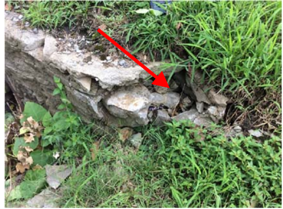
Failing Inlet Headwall
