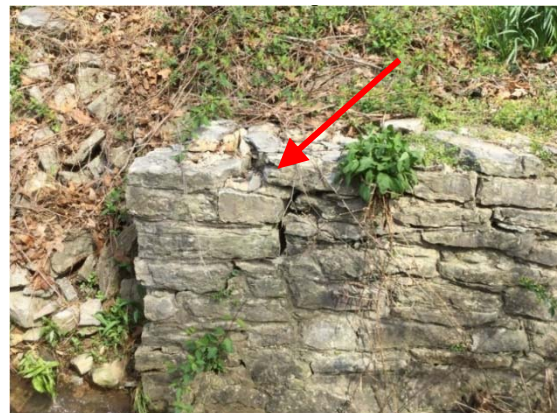
Failing Headwall
