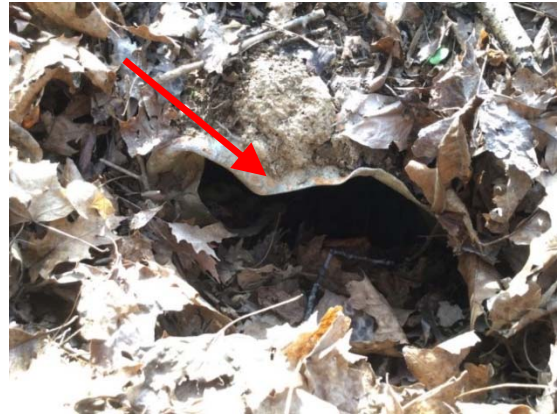
Crushed Pipe Inlet
