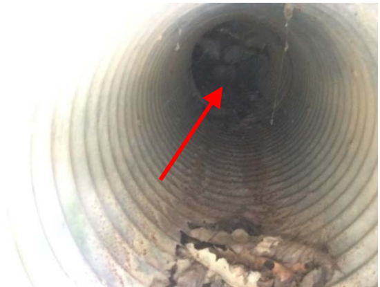
Crushed Pipe Inlet
