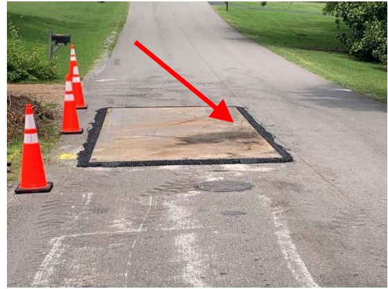
Roadway Failure w/ Steel Road Plate
