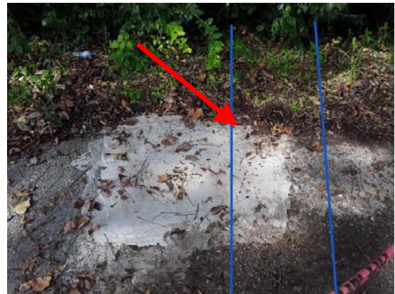
Patched Roadway Failure
