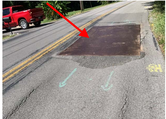
Roadway Settlement w/ Steel Road Plate
