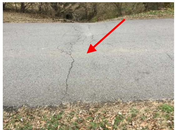
Section Loss & Pipe Collapse
