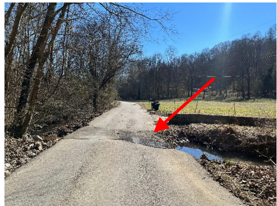
Pavement Settlement/Failure
