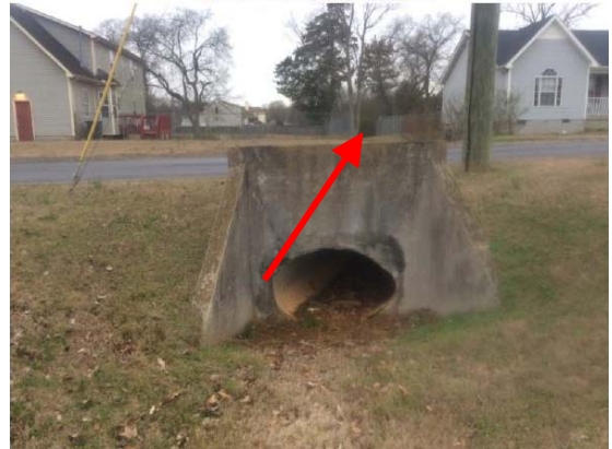
Partial Pipe Collapse
