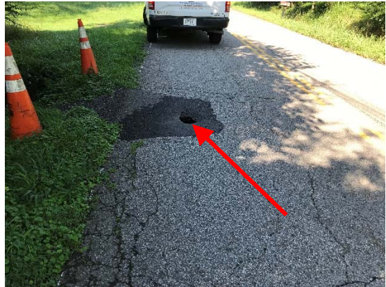
Roadway Failure w/ Steel Road Plate
