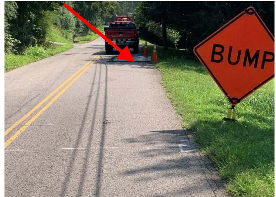
Roadway Failure w/ Steel Road Plate
