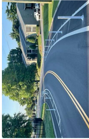
PROTECTIVE BARRIERS AND MARKED LANES
