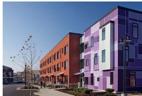
Ryman Lofts in Rolling Mill Hill
