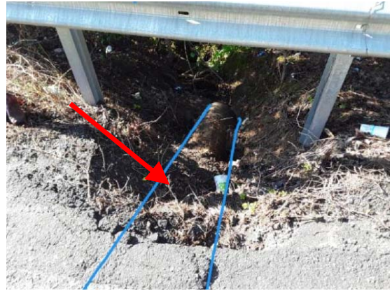
Embankment Failure
