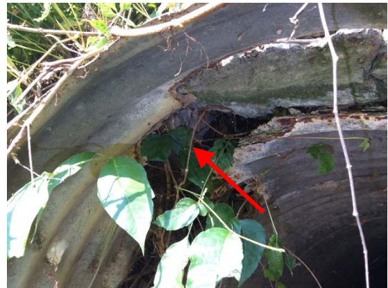
Erosion @ Inlet Headwall
