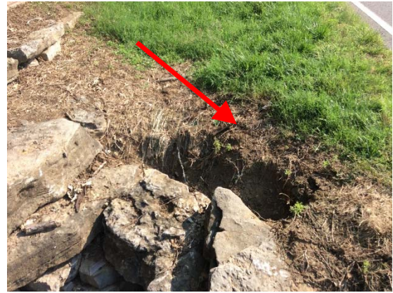
Erosion @ Inlet Headwall
