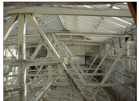
Structure for skylight inside Union Station on Broadway.
