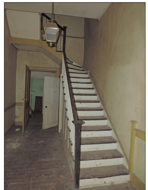
Staircase of the Hall-Harding-McCampbeell House at 305 Kent Road, prior to rehabilitation.
