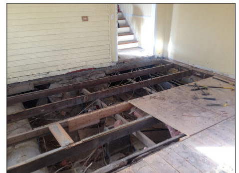
Wood floor replacement where the original floor did not exist.
