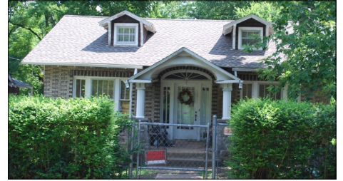
162 Kenner is a Colonial Revival style home in a bungalow form.
