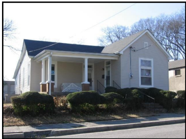
Gabled-ell at 1805 4th Avenue North.
