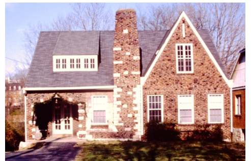
116 Kenner Avenue is an example of the Tudor Revival style.
