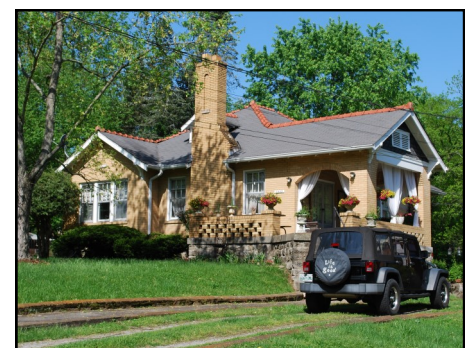
3509 Golf Street is one of the earliest homes constructed on this street in 1927. It retains its terra cotta ridge, a common feature in the district.
