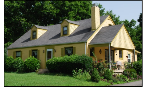
1121 Eastdale Avenue is an example of the Colonial Revival style applied to a Minimal Traditional residence.
