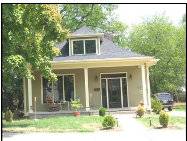
Hipped roof with full-width porch at 1706 5th Avenue North.
