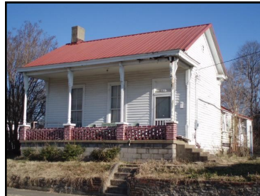
Side gable at 1810 5th Avenue North.
