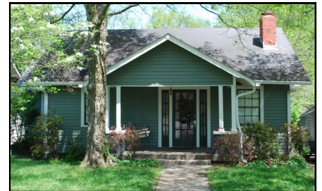
1127 McChesney is a good example of the bungalow form.
