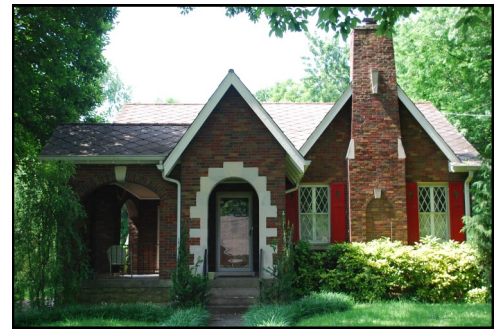
The Tudor Revival style is found at 1106 Riverwood Drive.
