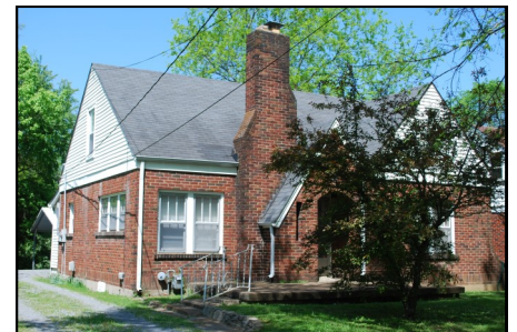
2312 Riverside Drive is a one and one-half story English Cottage constructed c. 1935.
