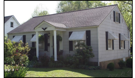
3518 Kennedy is an example of the Colonial Revival style applied to a Minimal Traditional residence.
