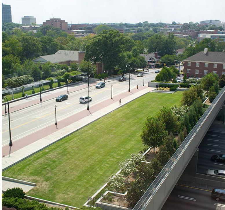
The 5th Street Bridge, Atlanta, GA
