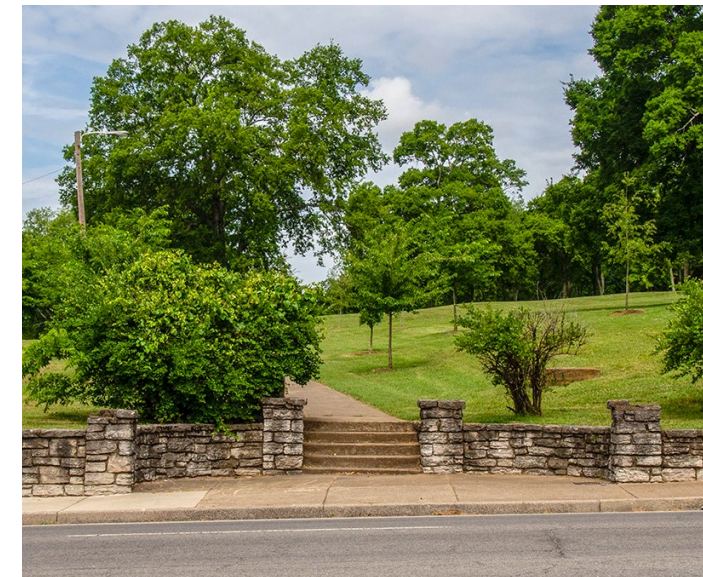
Reservoir Park Stairs and Walls
