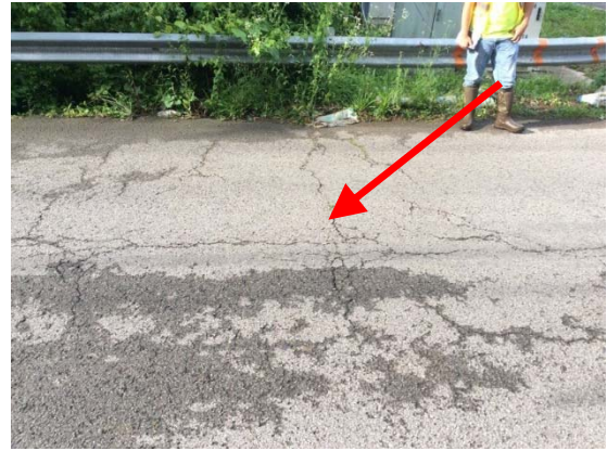
Pavement Cracking & Settlement
