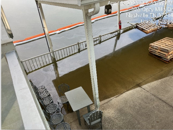
Photos of the Petroleum Containment/Absorbent Booms Deployed at Dock Sinking Fuel Spill
