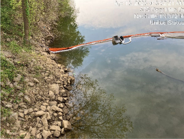
Photos of the Petroleum Containment/Absorbent Booms Deployed at Dock Sinking Fuel Spill
