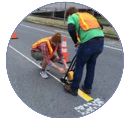
Temporary Reflective Striping
