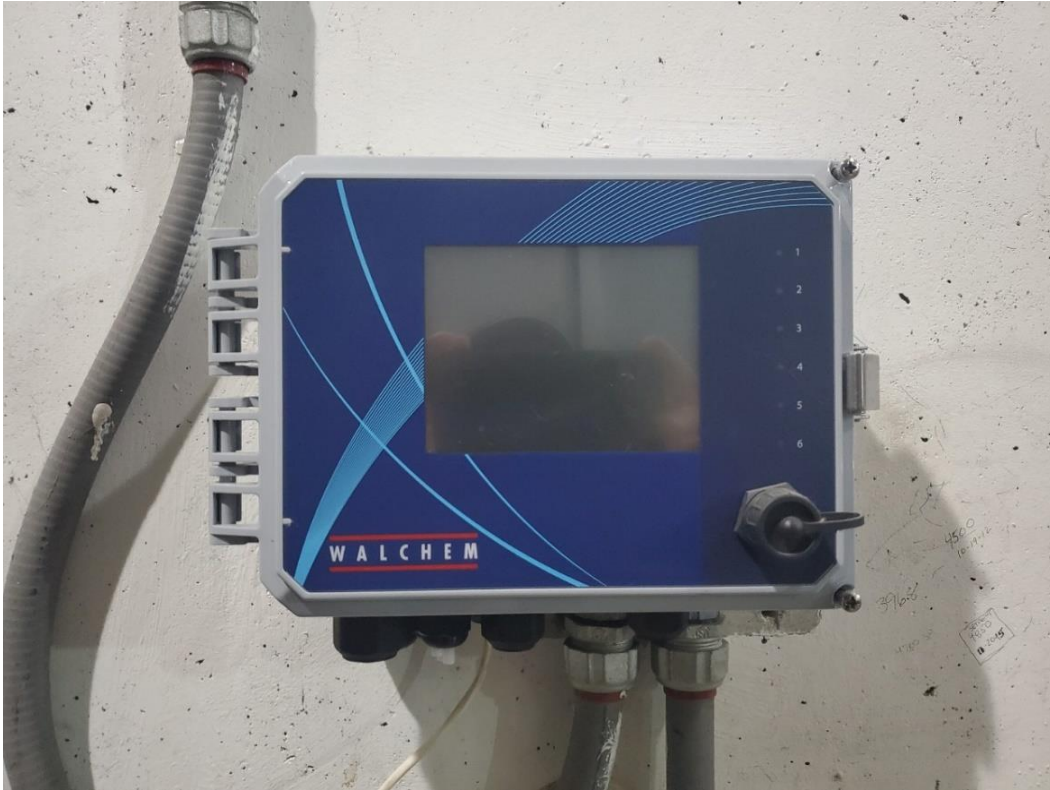
#1 Boiler Conductivity Controller Upgraded (new panel)
