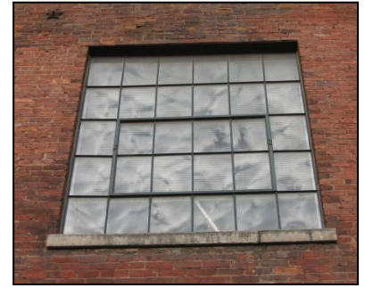
This historic metal window should be repaired as needed and retained.
