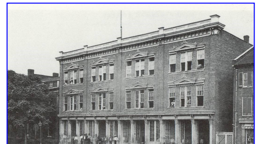
417-423 Broadway in 1864 showing the original cornice at the roofline and pedimented cornices over the windows. 615-862-7970
