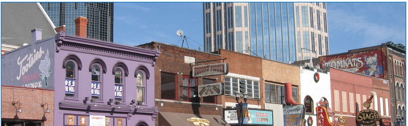
The flat rooflines of these buildings are typical of district buildings. If roof repairs or replacements are required, the historic roofline appearance should be retained.
