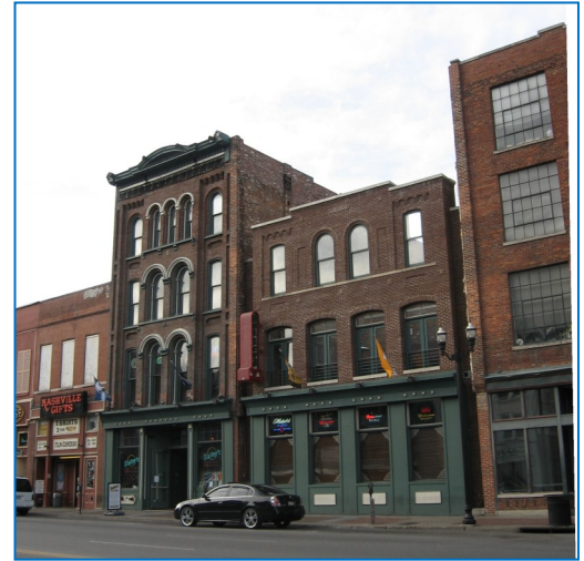
The infill building on this block appropriately maintained the established setback and rhythm of spacing.
