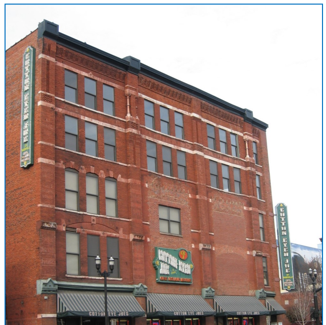
Property owners are encouraged to rebuild missing façade elements such as the bay windows removed on the second and third floors of 200-204 Broadway. 615-862-7970
