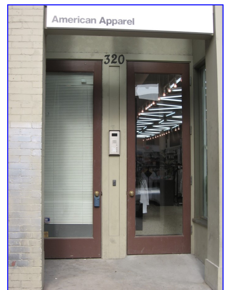
Appropriate modern doors at 320 Broadway.
