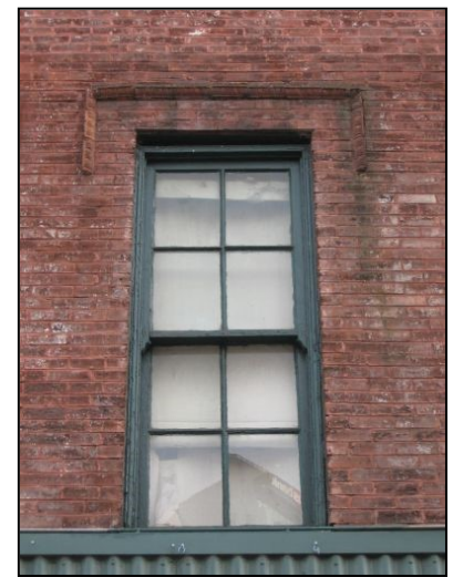
This modern replacement window is an appropriate design for this building and has a wood frame, clear glass panes, and a double-hung four-over-four configuration. 615-862-7970
