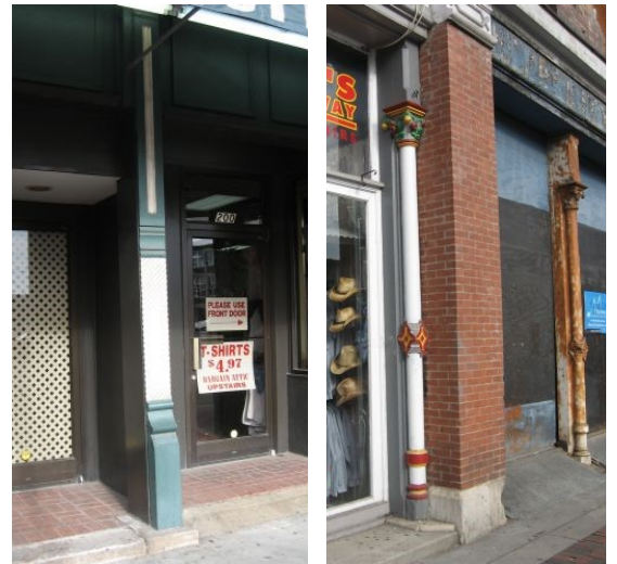
The cast-iron pilasters (left) at 200 Broadway are important structural and design elements to the building. The cast-iron columns (right) are historic and should be retained. The paint used on the left column is appropriate and a good maintenance measure. The column on the right awaits cleaning and painting.
