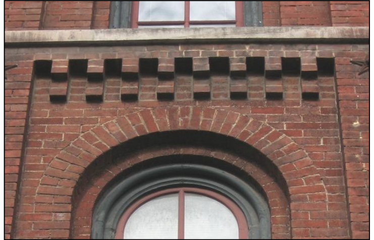
Decorative brick corbelling frames this window.
