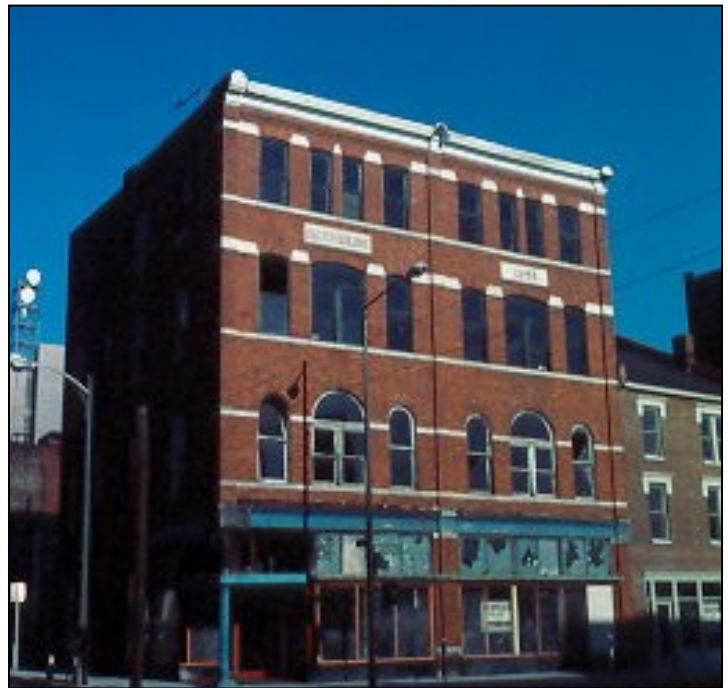
The Baxter Building before (above) and after (below) it was chemically cleaned to restore the original brick surface.
