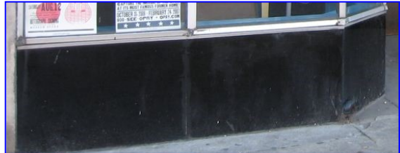
Both the tile-covered and the Carrara-glass-covered bulkheads above are historic. These materials should be retained and preserved. If needed, they should be repaired using materials that allow them to retain their historic appearance.
