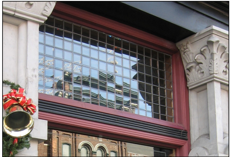
This modern transom on the Merchant's Hotel imitates multi-pane transoms of the turn of the century.
