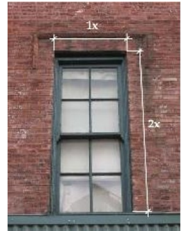
Appropriate proportions for upper-floor windows.
