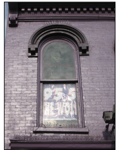
Original one-over-one arched window with sheet metal hood molding. Historic windows and window components should be preserved and retained.
