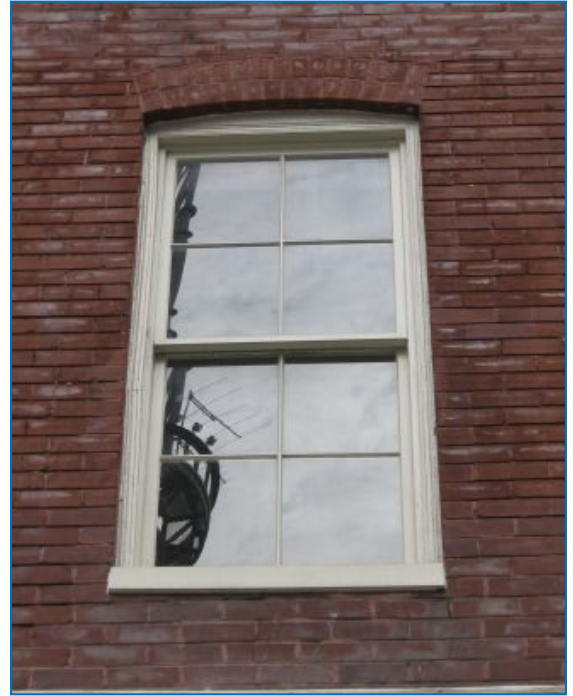
Appropriate modern four-over-four sash replacement window.
