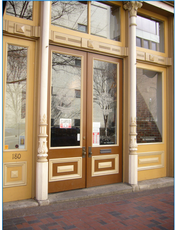
Historic transoms should be retained and preserved.
