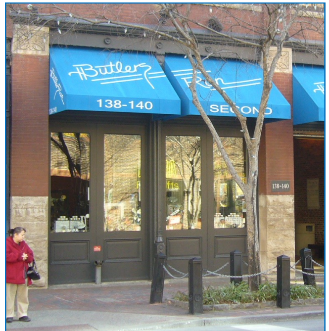
This modern storefront appropriately replicates the missing historic storefront through its incorporation of the typical storefront elements of wood-paneled bulkheads, and clear glass display windows with wood frames.
