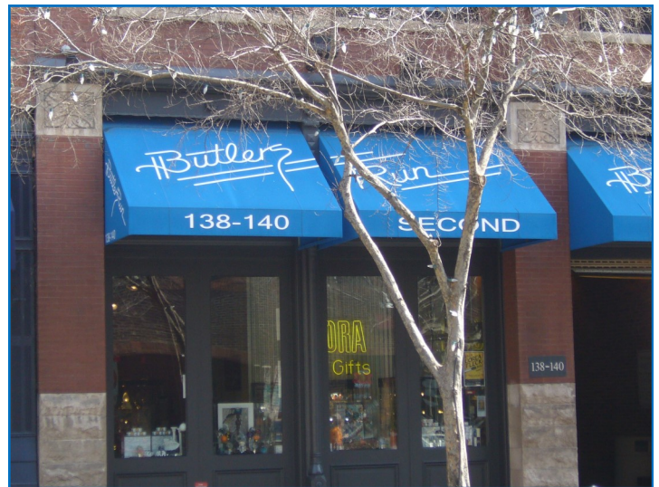
The placement, above the storefront and transom, and shed form of this awning are appropriate. Likewise, its opaque construction material is appropriate. As illustrated, awnings may include graphics or signage.
