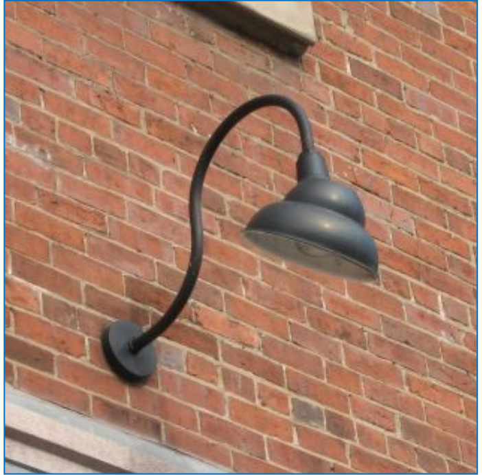
The simple design, inward direction of the light, and dark metal construction of this light fixture make it appropriate.
