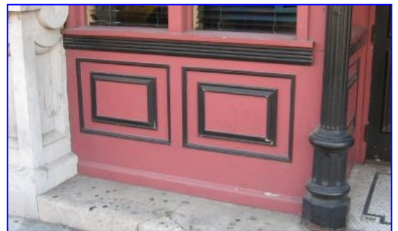
The painted, paneled wood is an appropriate modern bulkhead design.
