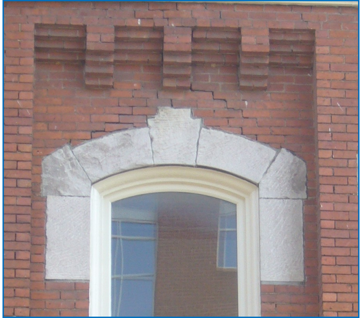
Decorative brick corbelling frames this window.
