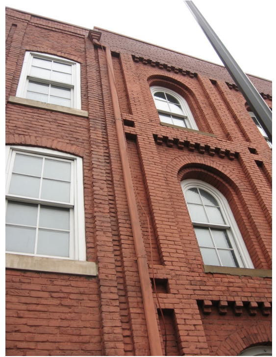
Downspouts on front or side facades should be painted to blend with the paint or masonry color.
