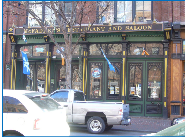
Original display windows should be retained and, if needed, repaired using materials that preserve their historic appearance.
