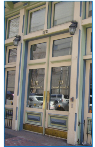
These and other historic doors should be retained. If repairs are needed, materials such as wood or wood epoxy should be used so that they continue to have their historic appearance.
