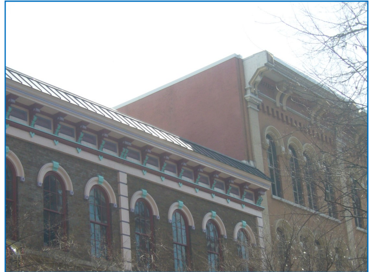
The roof shapes for new construction should mimic the roof shapes of existing buildings. On this block, as is typical for the district, appropriate roof shapes are flat or very slightly sloped and some have gabled parapet walls.
