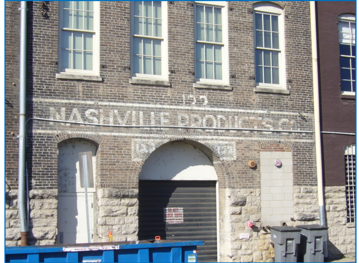
Original façade walls should be retained without the addition of balconies or other non-historic building elements.
