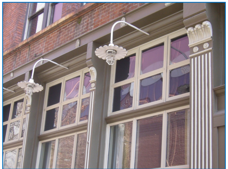
The simple, industrial design and inward direction of the light make this light fixture appropriate.
