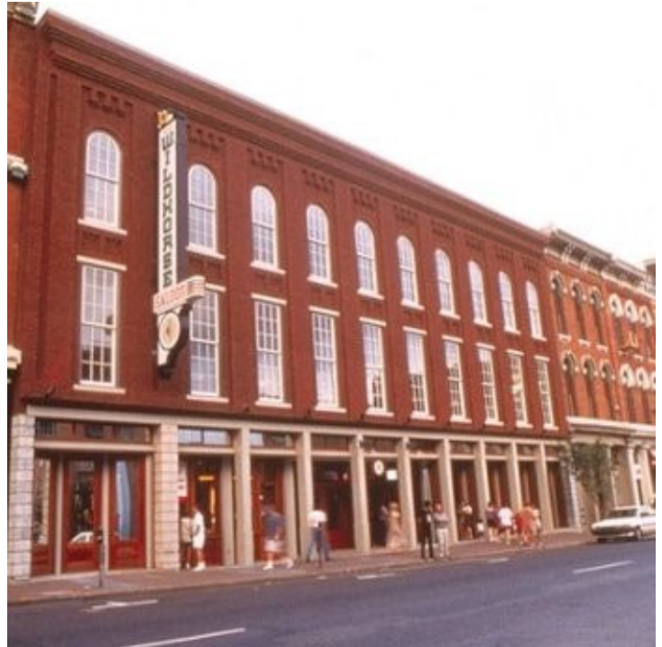
This building was reconstructed based on photographs.
