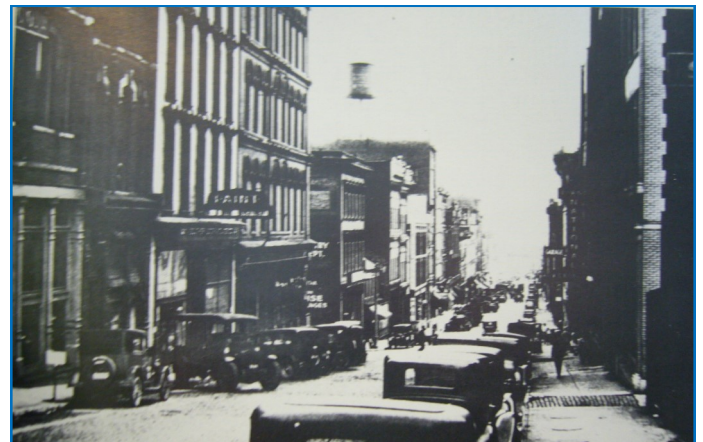
This view is from Church Street looking north on Second Avenue and shows how the automobile age of the 1920s started to change the look of Nashville.
