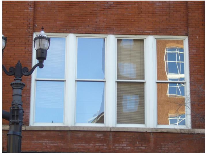
A one-over-one window design can be appropriate when the original grill pattern is unknown.
