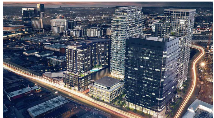
08G: Paseo South Gulch (Gulch South) presents a unified design concept in its relationship between the lower levels of new towers to the scale of surrounding historic buildings and outdoor spaces.
