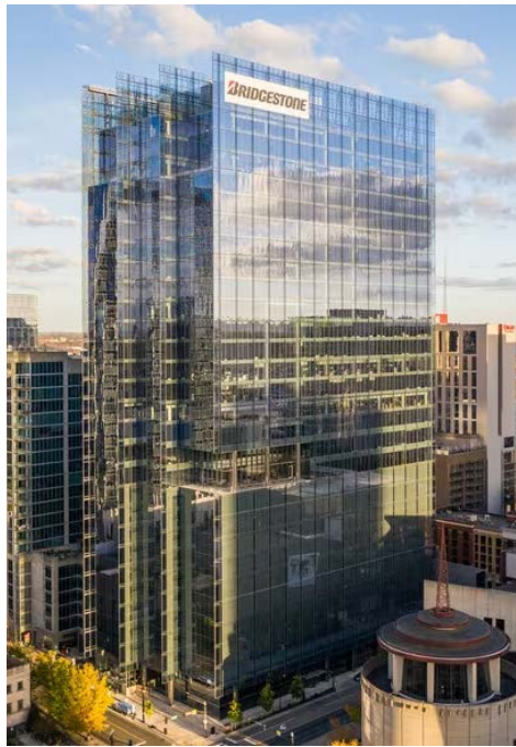
04F: Parking levels, at the Bridgestone Tower (SoBro) are screened from view with materials that fit seamlessly into the tower design.
