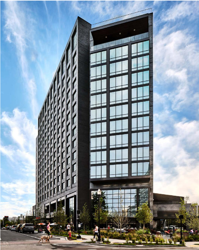
08C: The Virgin Hotel (Music Row) features a design that responds to its context at a major intersection. It presents a unified aesthetic between its lower levels and their relationship to the human scale and the upper floors, through clear massing, articulation, and fenestration.
