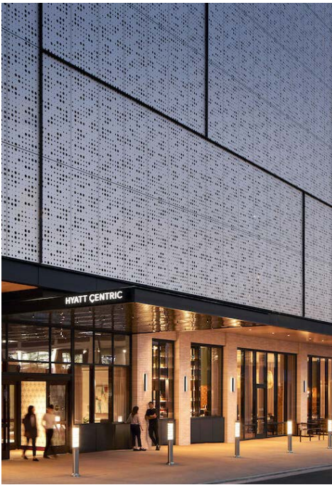
04E: A screening element at the Hyatt Centric (SoBro) features a low percentage of openings.
