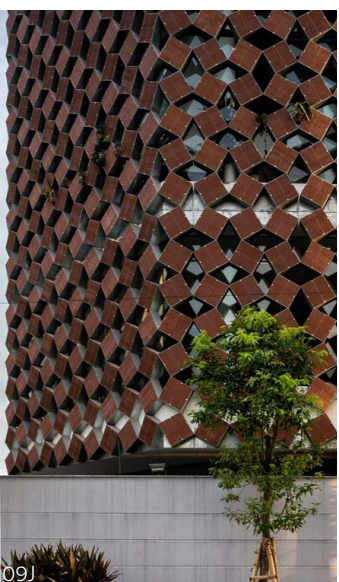
09B-L: Façade articulation can be implemented with different scales of granularity, responding to and maximizing on the inherent nature of the selected materials, and adding aesthetics and texture to the street wall. Performative systems that help reduce energy loads should be considered whenever possible.
