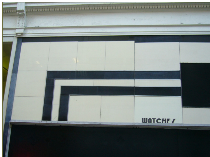
A portion of this storefront's original structural glass façade remains.
