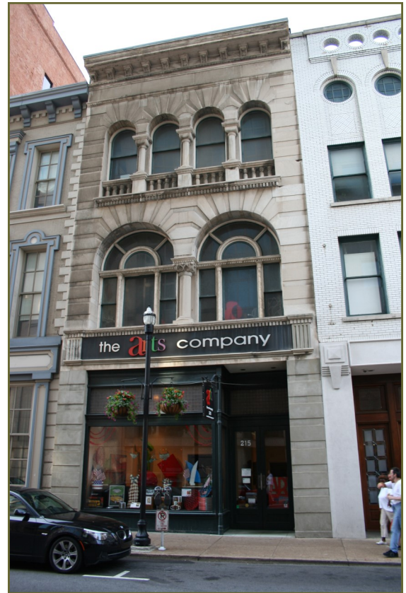
Original and early display windows like this at 213 Fifth Avenue North should be retained and, if needed, repaired using materials that preserve their historic appearance.
