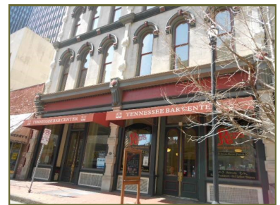
221 Fourth Avenue North was constructed in 1871 in the Italianate Commercial Style. While the storefronts have been altered, the façade retains its original upper floor details.
