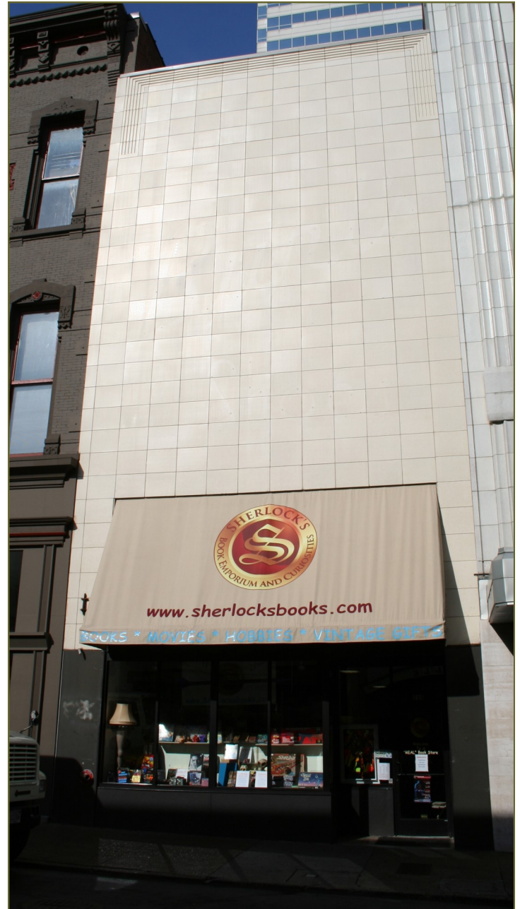
Property owners are encouraged to rebuild missing façade elements such as the windows and detailing removed at 235 Fifth Avenue.
