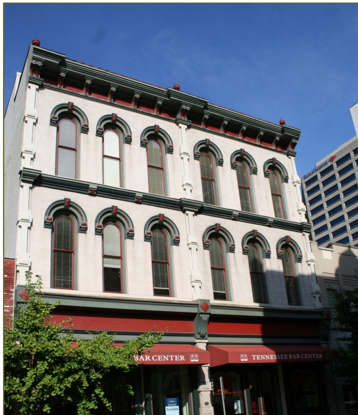
Original one-over-one arched windows at 221 Fourth Avenue North have sheet metal hood moldings. Historic windows and window components should be preserved and retained.
