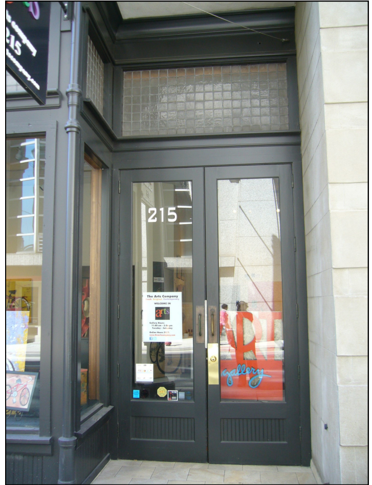
Historic transoms above windows and doors should be retained and preserved.
