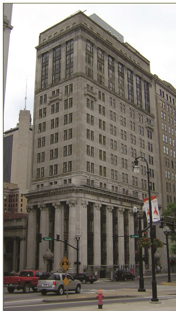
Historic buildings typically had some type of architectural detailing that broke the building into three parts: a base, middle and cap.
