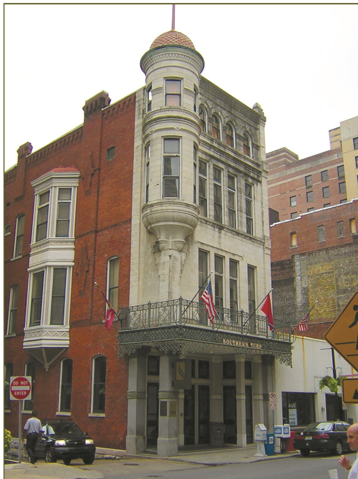
Character-defining features of the building at 224 Fourth Avenue include the corner turret, side bay window and metal canopy.
