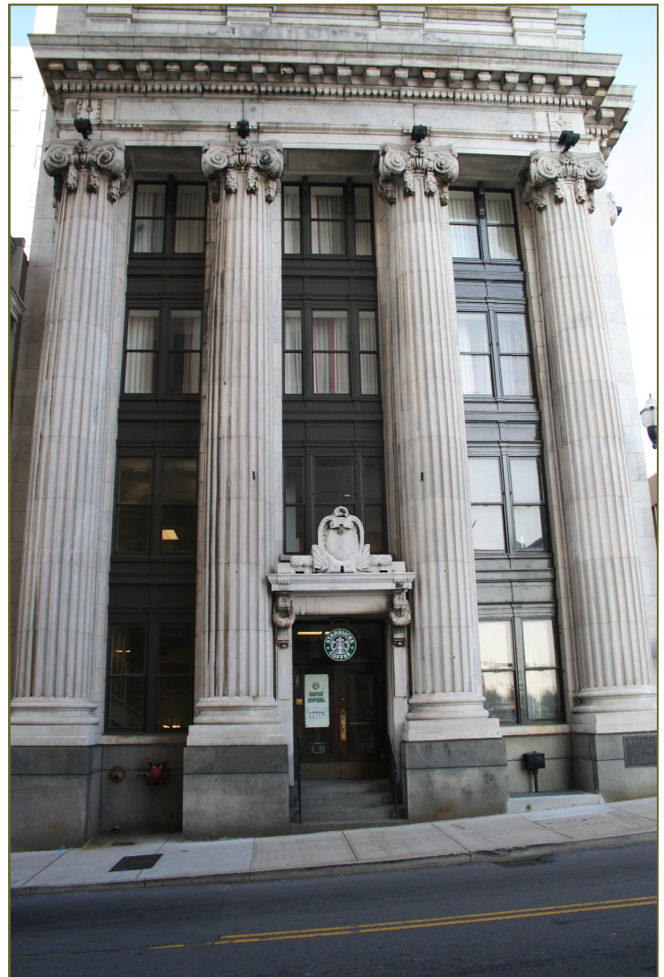
The stone columns at 227 Third Avenue North are an important design element to the building.
