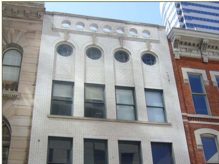
When the original window pattern is unknown, a simple one-over-one design for replacement single or double-hung windows is an appropriate choice.
