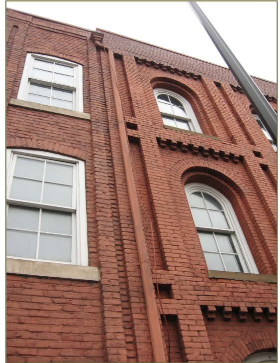
Downspouts on front or side façades should be painted to blend with the paint or masonry color.
