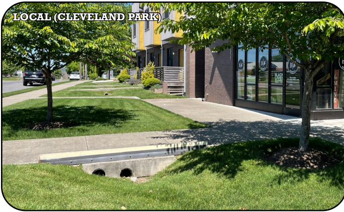
Stormwater management underneath sidewalk
