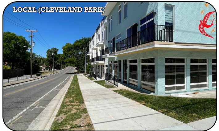
Wide buffered sidewalk
