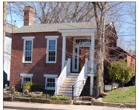
One of Germantown’s oldest residences (c. 1840) on Fifth Avenue North during a renovation.
