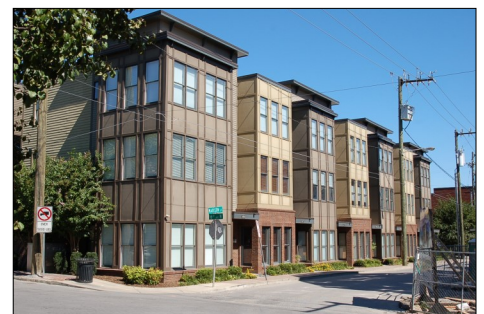
Infill at Sixth Avenue North and Madison Street.
