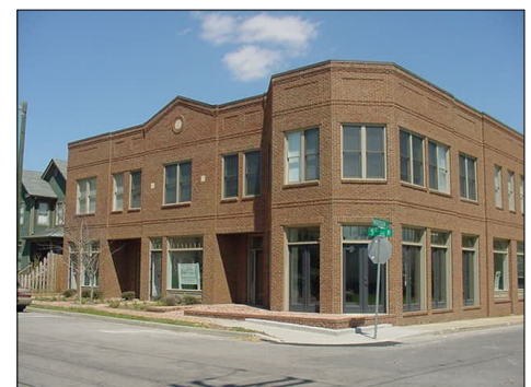
Infill at Fifth Avenue North and Madison Street
