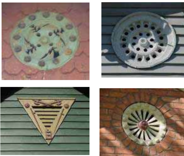
Examples of historic attic ventilation grilles.
