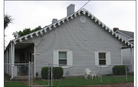
Historic duplex at 1315 6th Ave North
