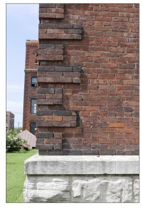
Original masonry details such as the corbelling on the corner, should be retained.
