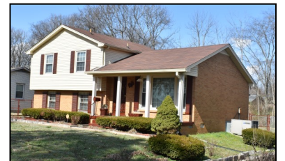
3822 Cravath Drive is an example of a one and one-half story split level form.
