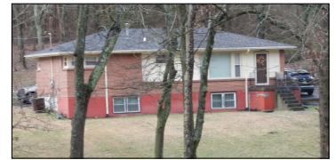
2512 Shreeve Lane is an example of a Split Form.
