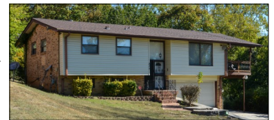
825 Youngs Lane is an example a cantilevered second level.
