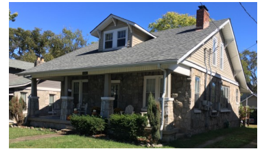
This building is an example of a one and one half story building. A "half-story" means that the upper level space is fully under the roof and often evidenced by a dormer or window in the gable field. This building has a gabled roof dormer and windows in the side gable field on the 1/2 level.
