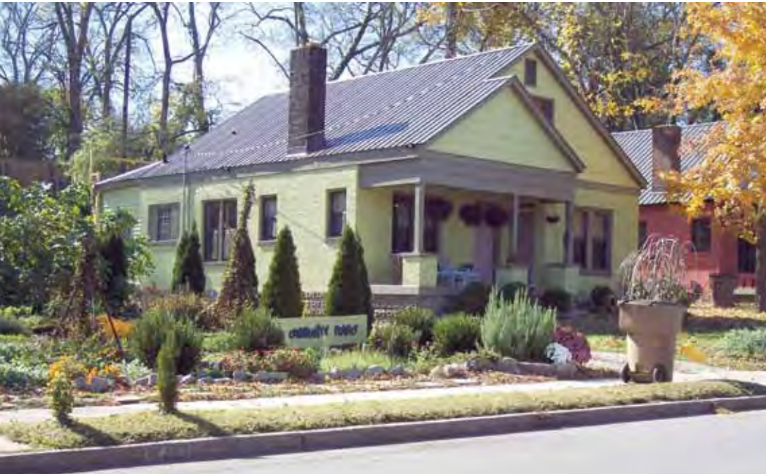
Historic homes in the neighborhoods flanking the Fourth Avenue South and Eighth Avenue South corridors have attracted new residents.
