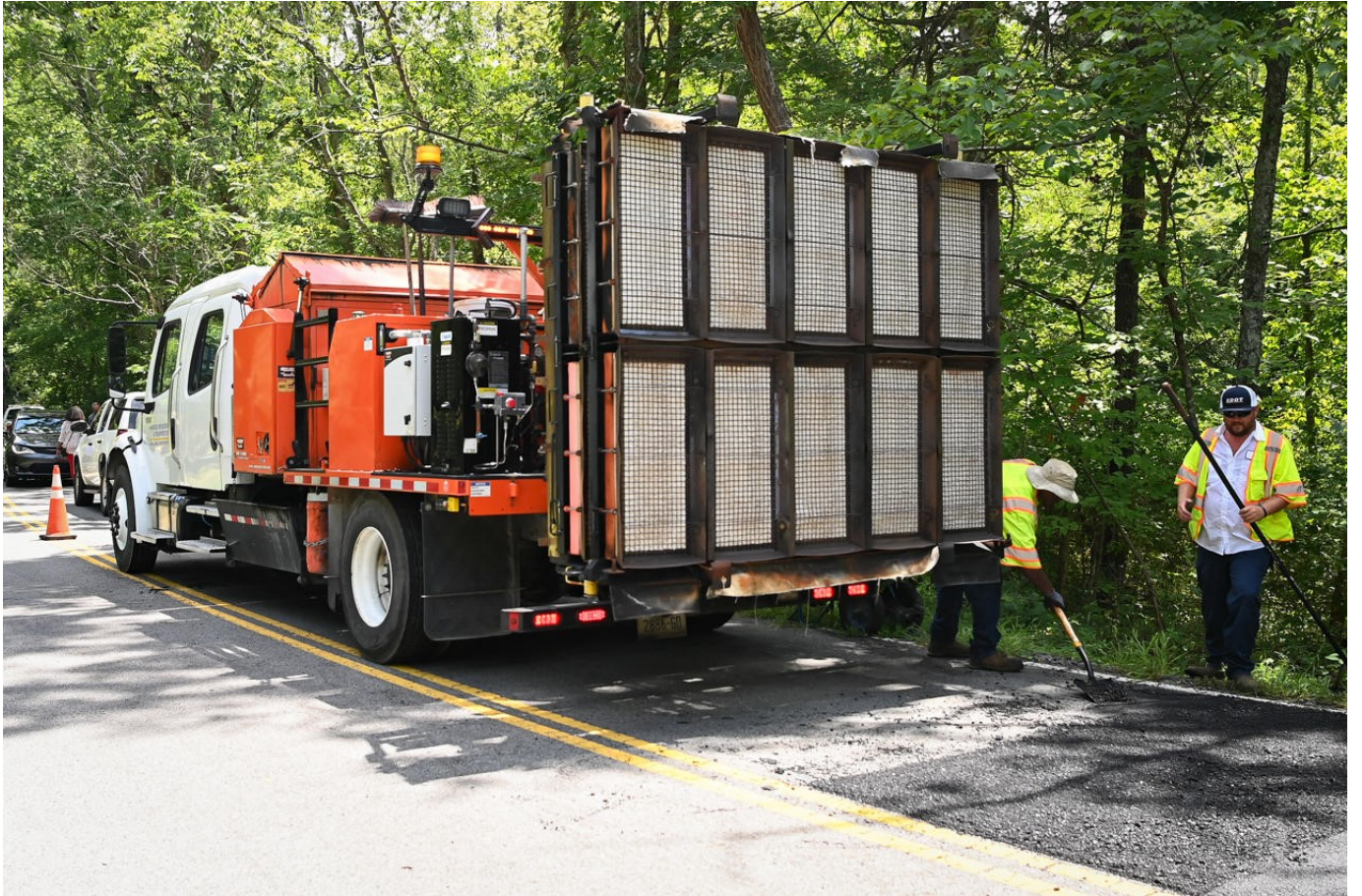
Photograph courtesy of the Mayor's Office
